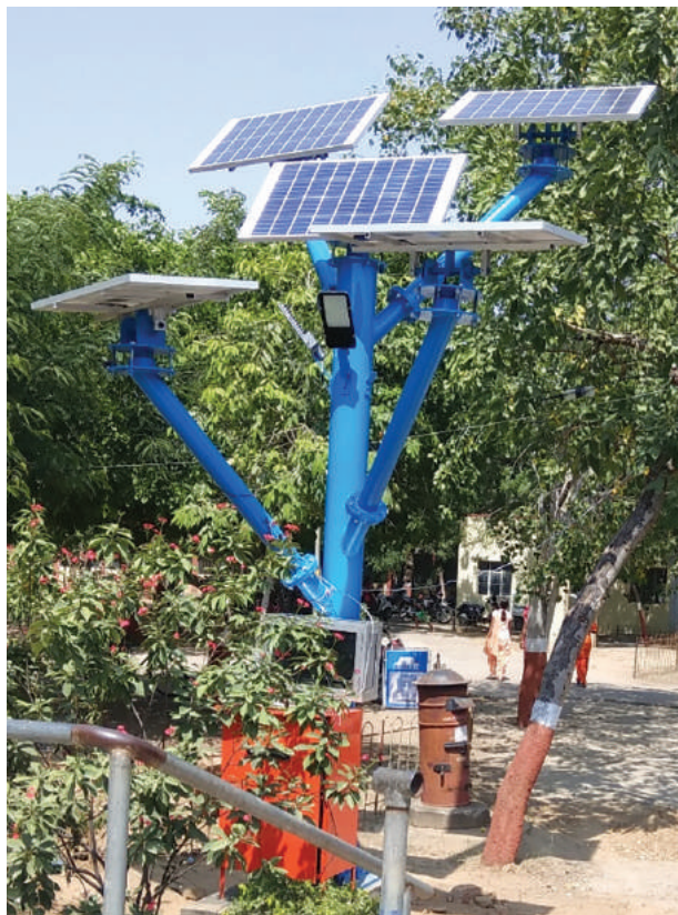
500 W solar tree installed at CSIR-CEERI, Pilani
