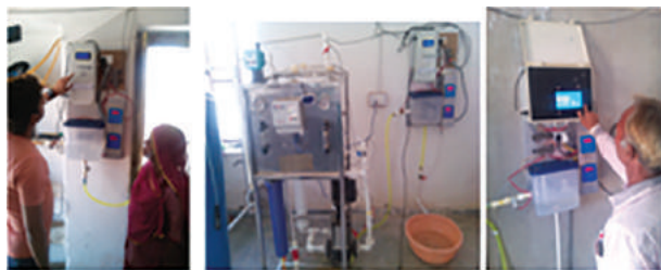
Field installation of RO status monitoring system
